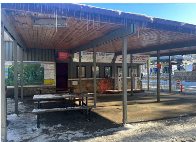
Figure 5 Note the general deterioration of the timber ceiling lining to the awning. Source: Kosciuszko Thredbo Pty Ltd, 08.08.23
