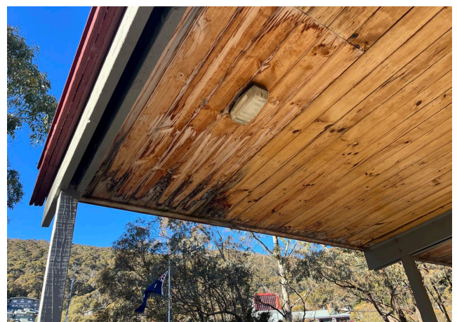
Figure 6 Northeast corner of the awning, note the deterioration of the timber ceiling lining. Also note the previous area of the lining that has been patched. Source: Kosciuszko Thredbo Pty Ltd, 08.08.23
